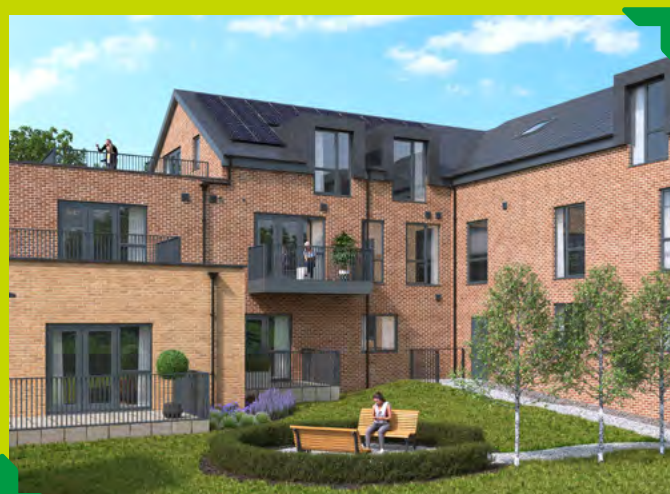
Solar panels at Westcliffs, Southend
